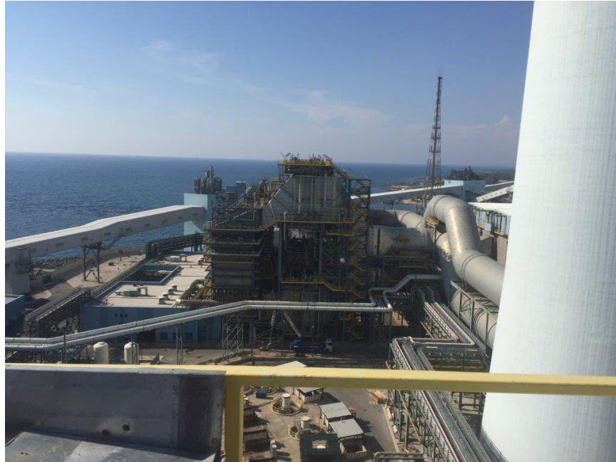
Figure 3: Side view of a tubular flue gas cooler.
